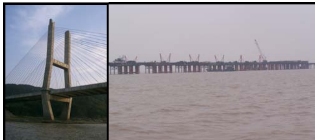
Fig. 8 Poyang Lake bridge and another bridge under construction nearby
