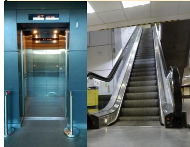
Lift and Escalator Installation
